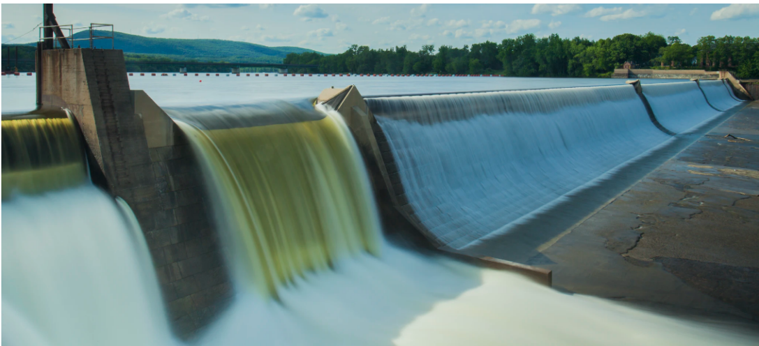
Holyoke Dam: Powering Hazen Paper with Hydropower
