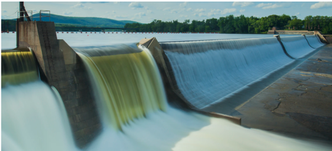
Holyoke Dam: Powering Hazen Paper with Hydropower
